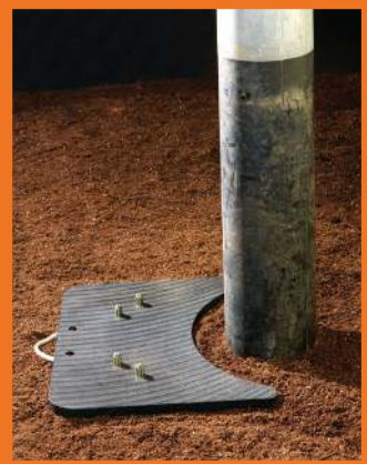
Place pole puller pad around the pole.
