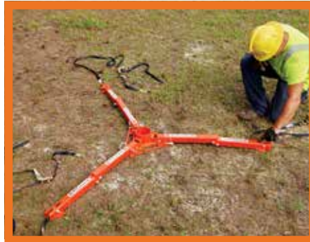
Position auger stand, remove locking pin and extend arms
